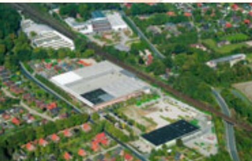
Since 1958 Production site in Hude, near Oldenburg
