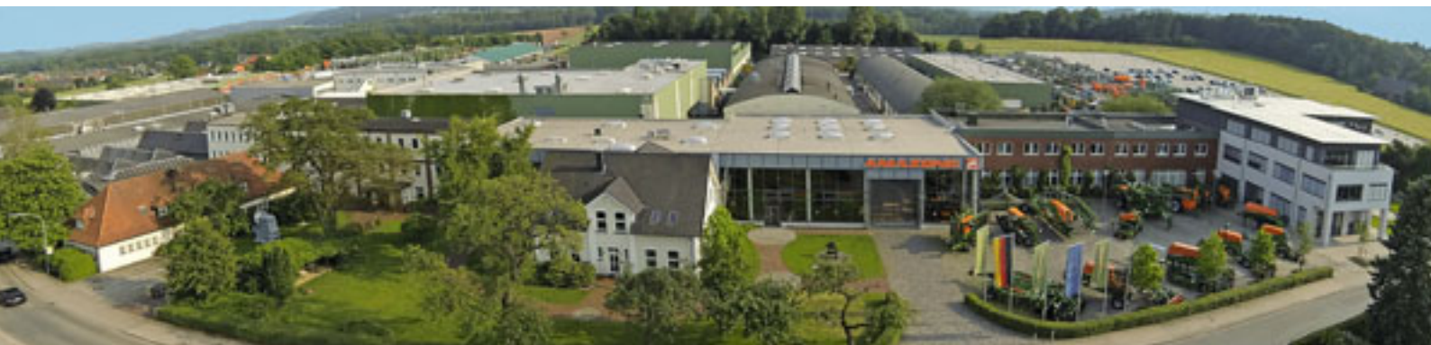
Headquarters in Gaste near Osnabrück
